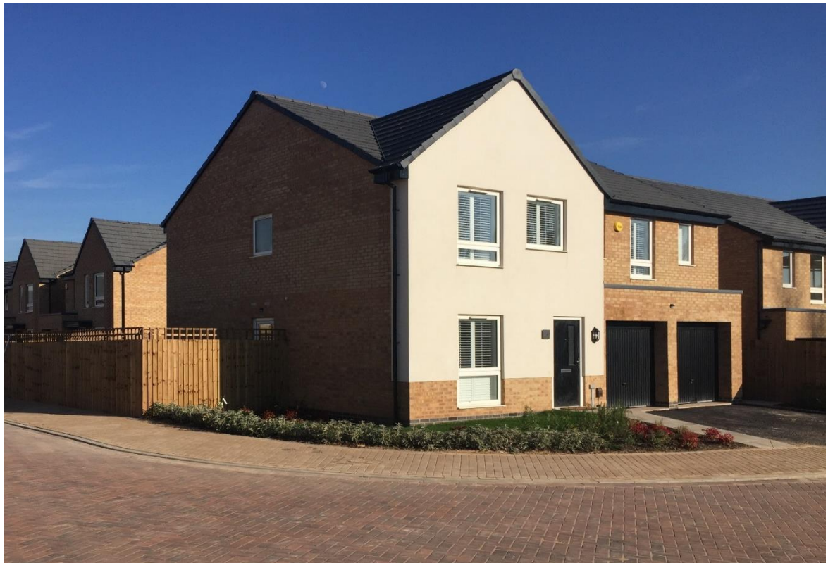
Photo new housing Gedling Colliery/Chase Farm
